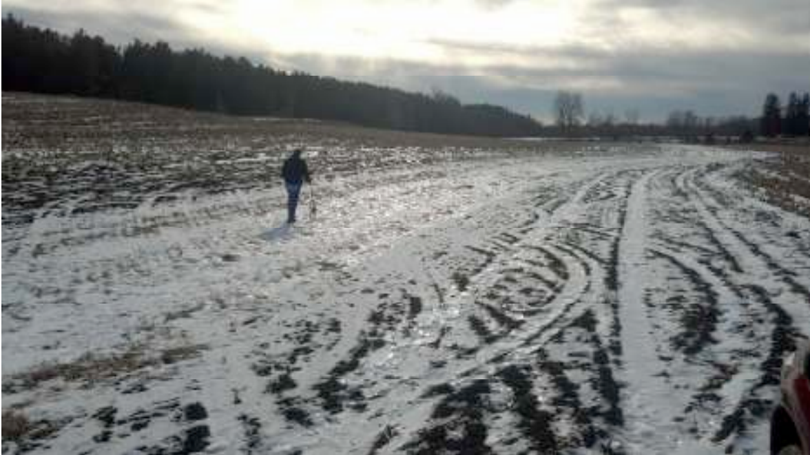
Dotolo Waterway Project – Pete Young measures and inspects the recently installed Dotolo grassed waterway in Scandia. The project was completed in December of 2011.
