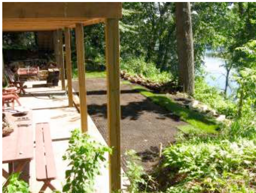
Mary Tilly Project – photograph shows the grass pave area adjacent to the river bluff.
