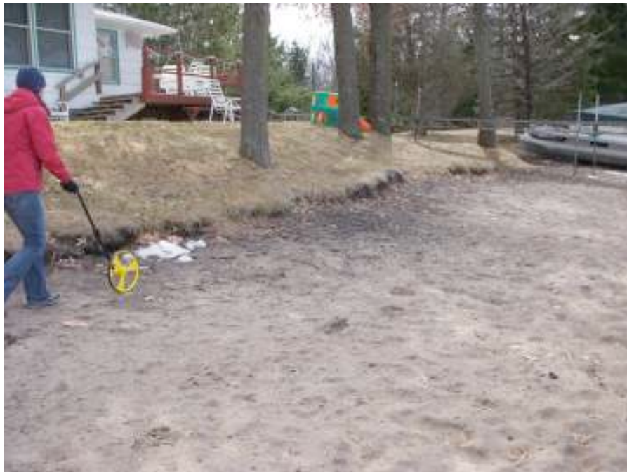
Mary Trost Property – Tara Kline takes a field measurement at the Mary Trost shoreline site in preparation for creating the group a final design. The shoreline planting will be installed in the spring of 2012. Erosion control features were installed in the fall of 2011.
