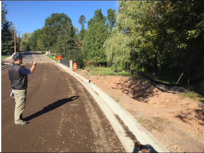
District Engineer inspects bio-filtration practice
